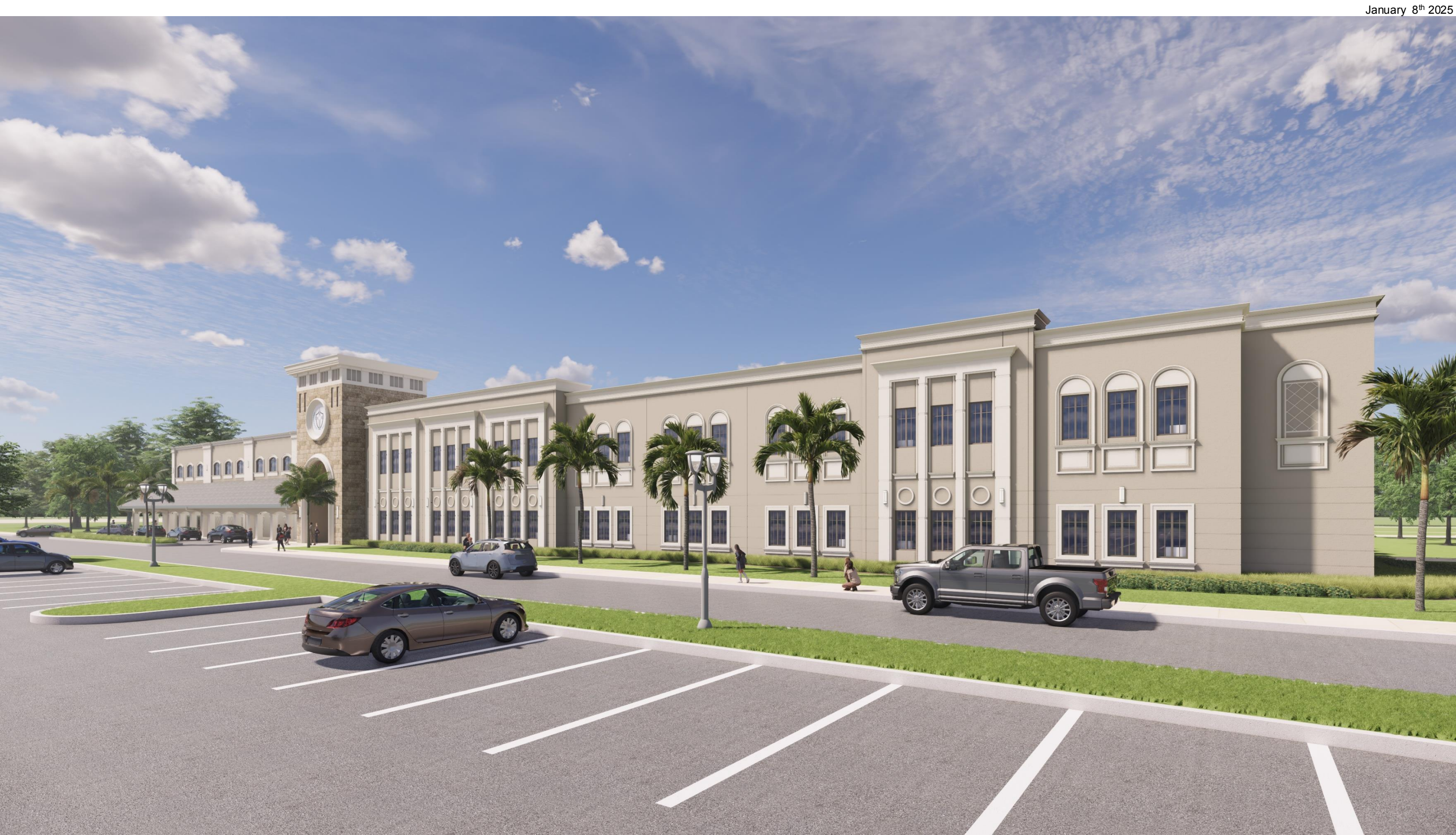
Phase I - Classroom Building 1A
